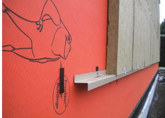
Figure 6: An example of a properly designed and installed rain screen. Note the unimpeded drainage cavity.
